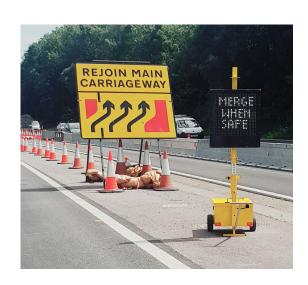
When there is no works traffic merging, after a set time, both signs revert to a blank display, maximising reliability by saving battery life.
